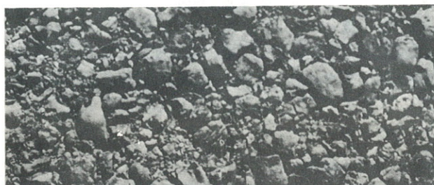
Close-up of lightweight seal coat after three years service
