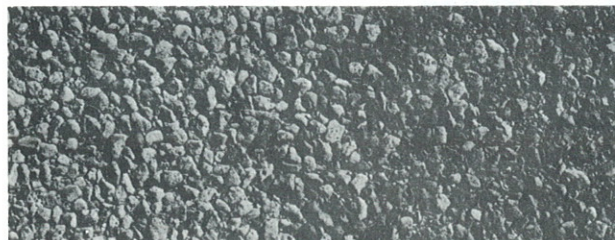
Lightweight aggregate seal coat still highly textured after six million vehicle passages-(1 2-inch top size materials)
